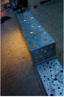
Praza Rei de Viana refurbishment
