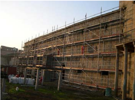
San Clodio monastery refurbishment
