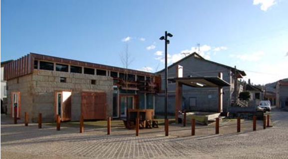
Library and public washing place refurbishment in Leiro
