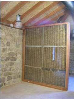
Mosteiro restaurant refurbishment
