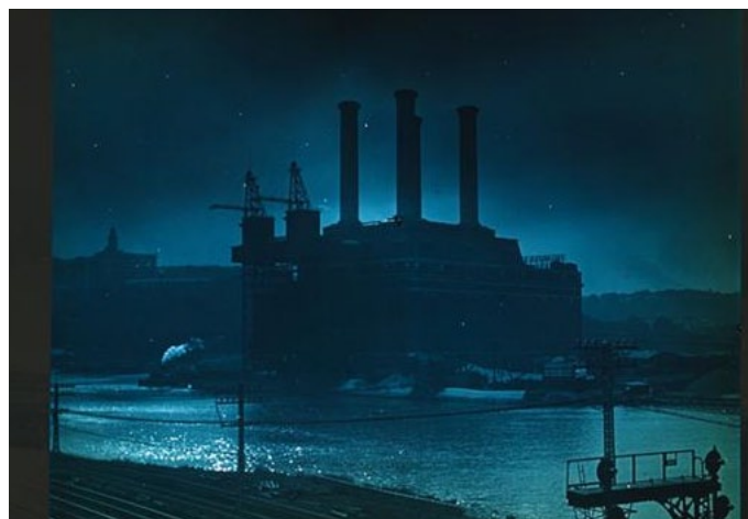
Sherman Creek, Energy Plant, 1914
