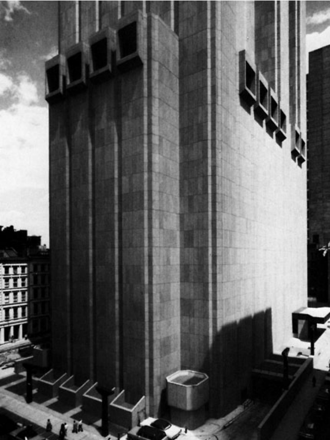
ATT, Long lines building, NY, John Carl Warnecke and Assoc 1966-72
