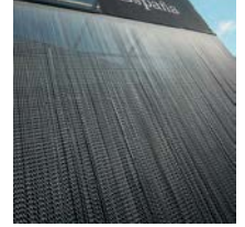
SOUND On the facade we opt for a metal curtain that informs about wind or rain through sound of its movement.
