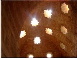
LIGHT-TEMPERATURE The windows are placed in higher positions in order to introduce daylight and sunlight.
