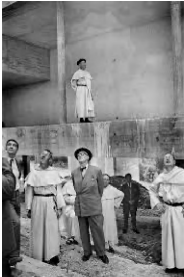
Le Corbusier, during La Tourette construction site, 1959. René Burri.
