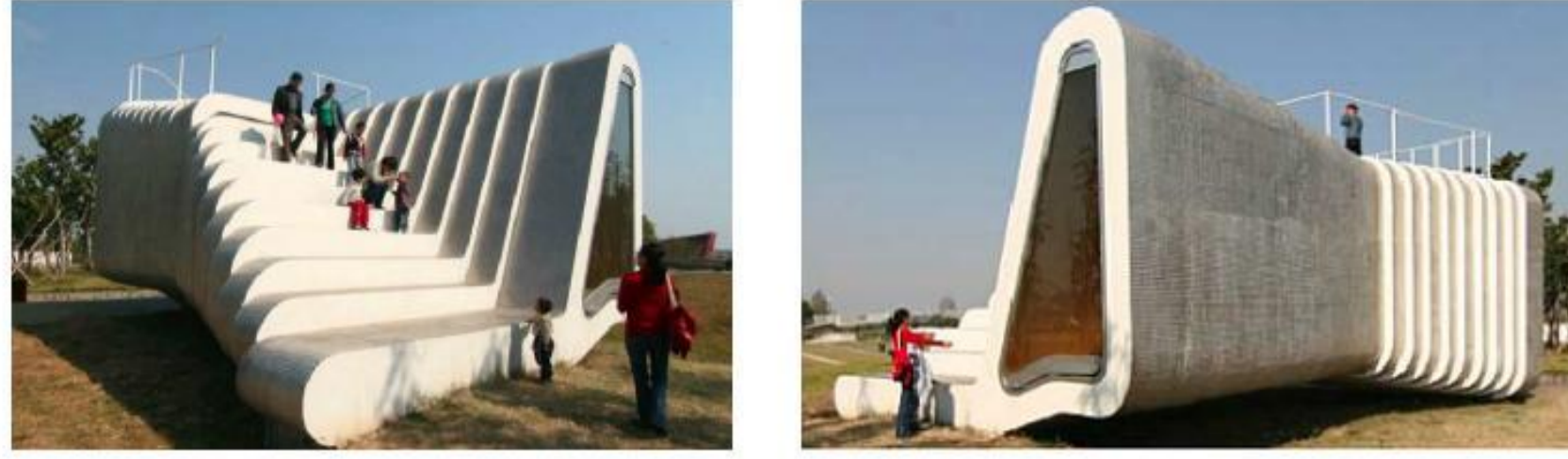
MULTIMEDIA PAVILION, JINHUA ARCHITECTURE PARK, JINHUA - CHINA (2007). ERHARD AN-HE KINZELBACH
