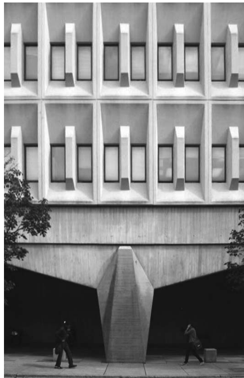
Becton Engineering Center
