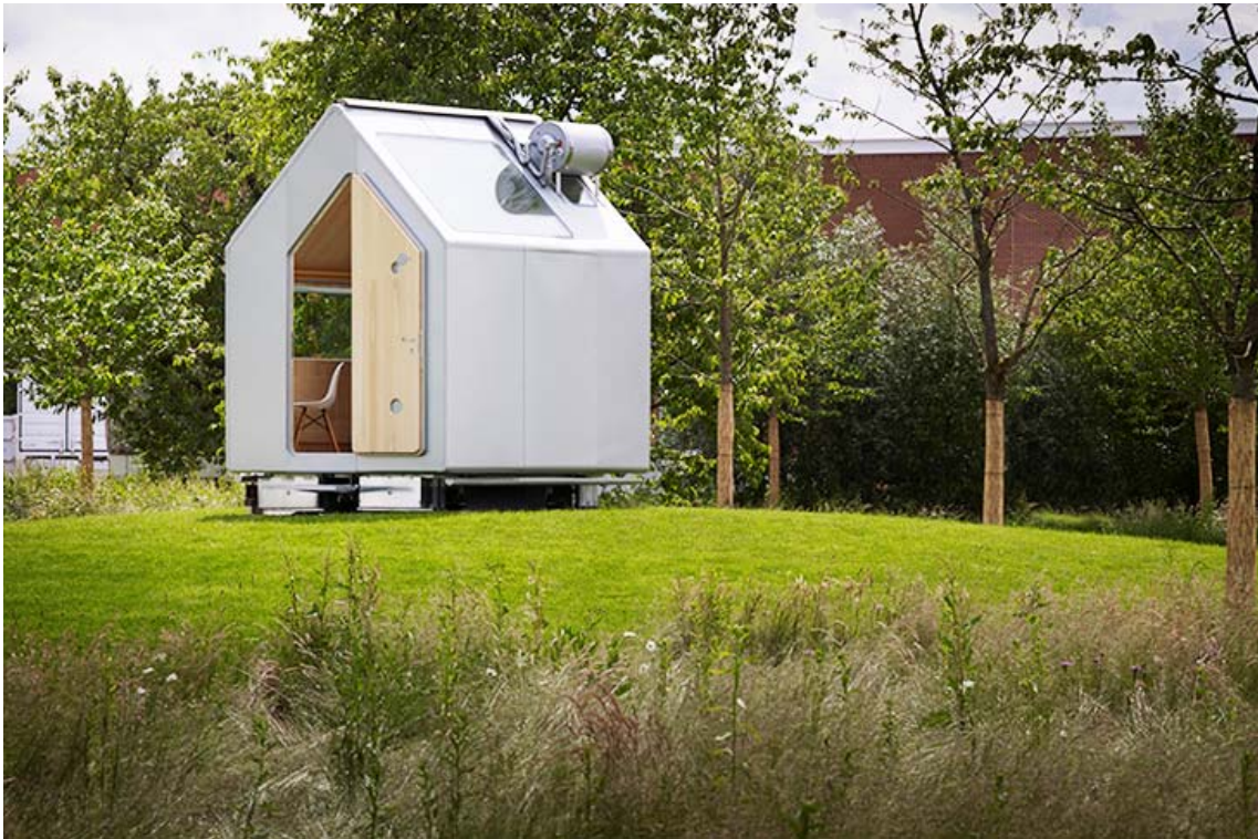
15. Cabanon de Renzo Piano, Vitra Campus, Alemanha. Fonte: http://inhabitat.com/renzo-pianos-tiny-diogene-hut-is-an-off-grid-shelter-for-one-person/vitra-campus-renzo-piano-pavillion-2/
